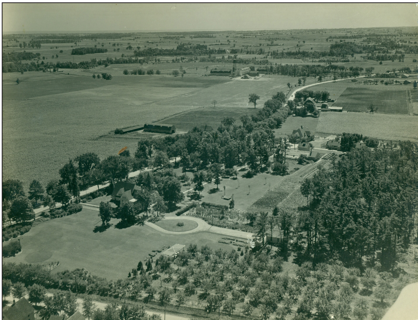
Aerial view of the entire Pinehurst farm looking south southeast toward the signature dairy barns taken prior to 1942. What is now Highway 32 is the road at left. Highway 28 does not yet exist—it later bisects the property. Today's Pine Haven Christian Home would be situated in the center of the image in the farm's extensive orchards.
