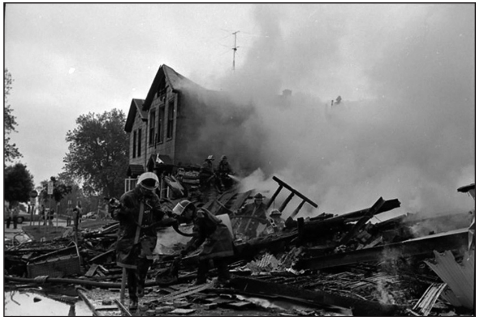
The aftermath of the Sheboygan Glass blast has firemen searching through debris and attacking hotspots. (Looking east toward Sixth Street.) More than 50% of the building was destroyed making it impossible to rebuild on this site according to changes in zoning laws. The company would need to move to an industrial park. In the short-term the company opened offices in the Motor Transport Terminal at Seventh and Jefferson.
