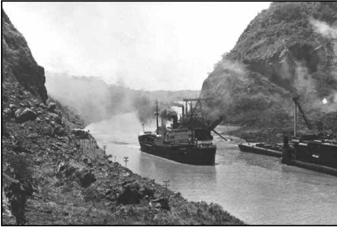
SS Ancon, the first ship through the newly opened Panama Canal in 1914, (U.S. Army Core of Engineers image) public domain
