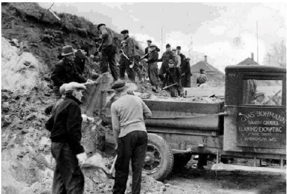
Work crews are removing the bluff just south of North Point in readiness for the creation of the new Broughton Drive. Charles Bohmann Sand & Gravel is taking away the fill.
