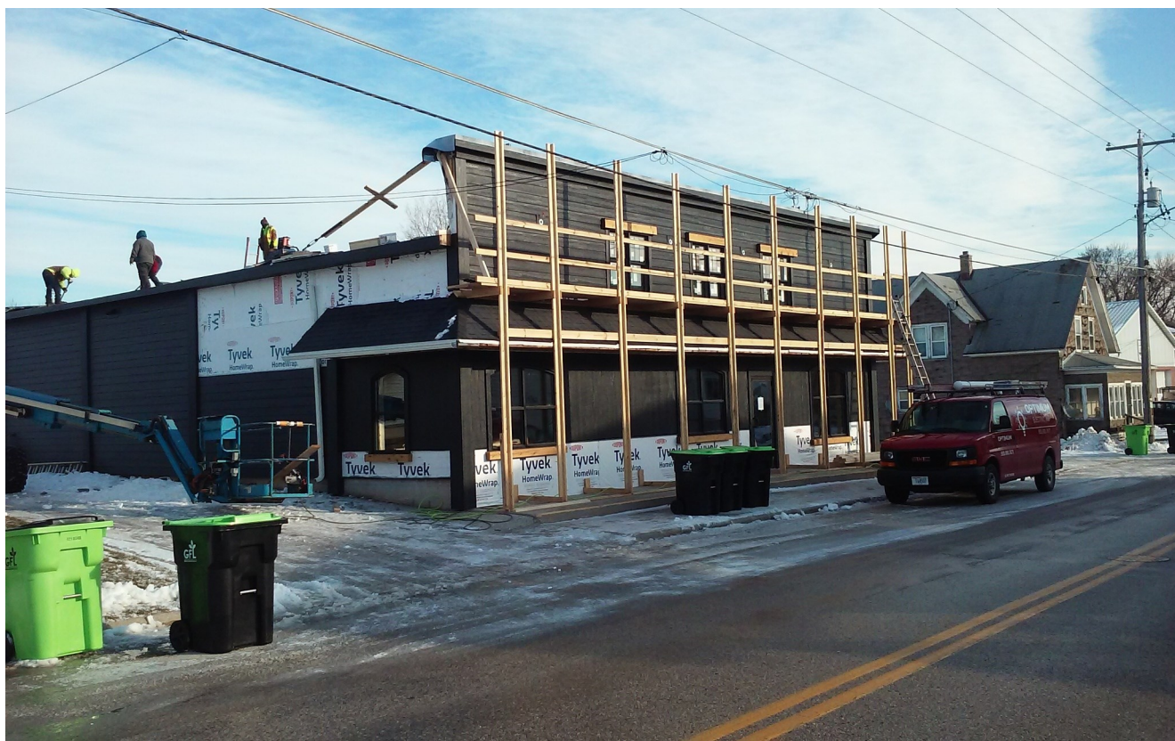
Neumann Plumbing & Heating Renovation-2021
