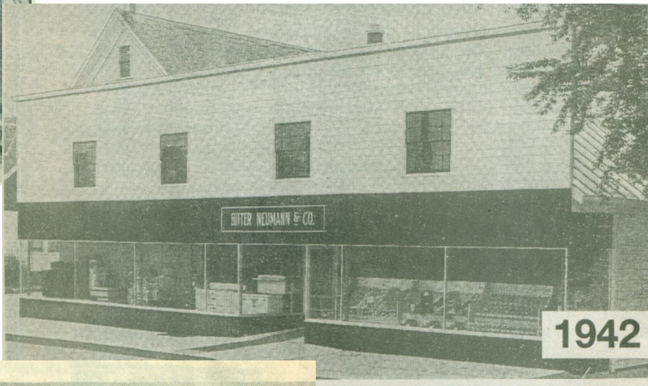
Millersville Store Remodeled 1942
