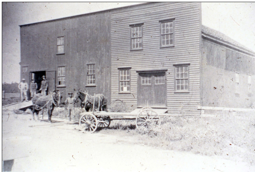
Schorer's Blacksmith Shop [ca. 1902]
