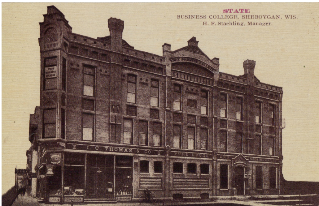
On April 11, 1887, the newly formed State Business College held its first class on the third floor of the new Zaegel Building on the southwest corner of North 8th Street and New York Avenue in Sheboygan. It was here that many Volga Germans went to night school to learn English.
